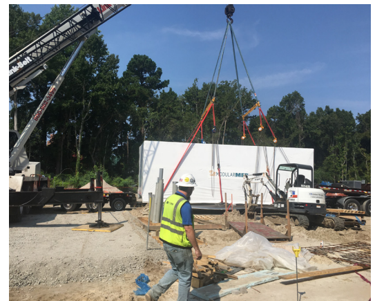
Receipt of prefabricated electrical rooms
