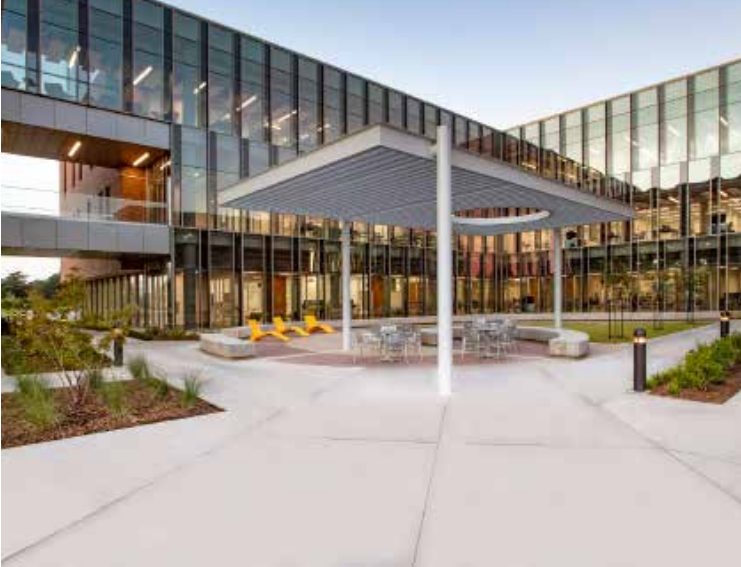
Tarleton State University • Engineering Building Stephenville, TX
